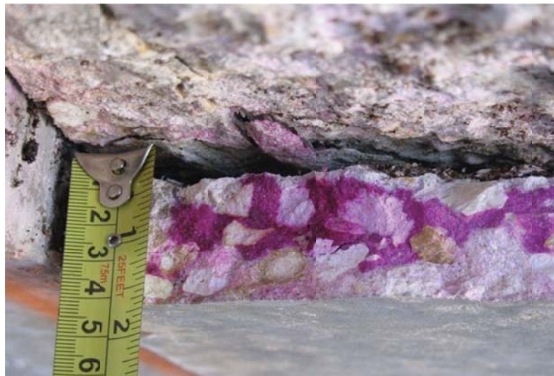
Figure 2.7 - Field exploration for carbonation detection
