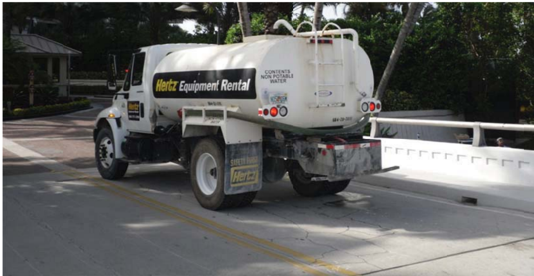
Figure 3.18 - Load truck for load testing
