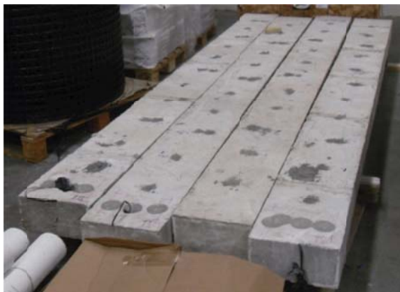
Figure III.D.1 - Visual inspection Beam B0 to B4 before corrosion
