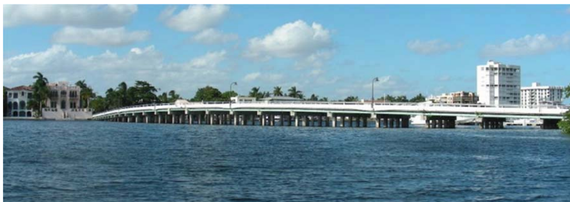
Figure 2.2 - Fair Isle Bridge from South-East direction
