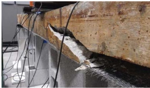
(c) concrete cover separation B3
